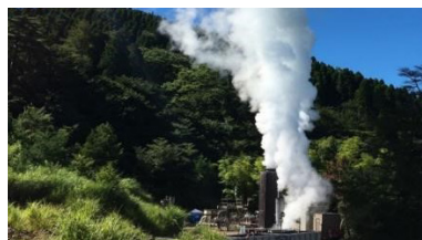
Geothermal power generation facility in Minami-Aso Village, Aso-gun, Kumamoto Prefecture
