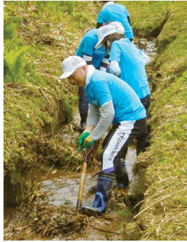
Employee volunteers removing mud from side ditches
