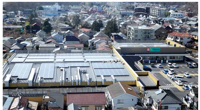
Photo provided by: Inageya Co., Ltd.
